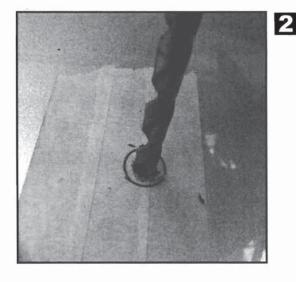
Control drilling position and rework, if necessary. Drill holes on Ø7mm and remove the masking tape. Before installing, control the threads in the feet to be free of dirt, if necessary with the enclosed screws.
